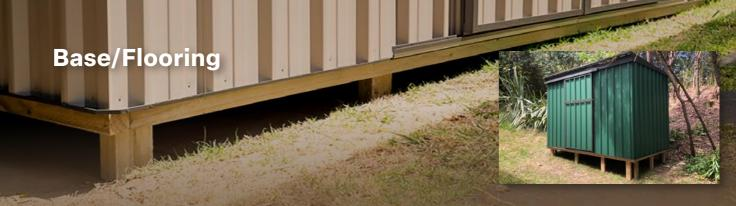
Your shed can be built directly onto lawn, concrete or decking. Our professional installers will make sure your shed base and floor is secured and level on your site using H4 treated timber and 18mm plywood flooring. A steel channel is wrapped around the base of the shed which the Colorsteel cladding is secured into. The cladding falls below the plywood floor level ensuring that the shed stays watertight and secure. Water easily flows away from the channel ends.
